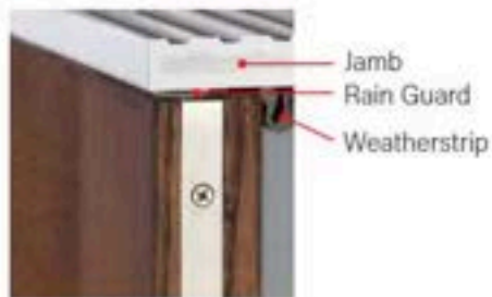
Top of door; exterior view.
