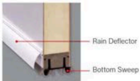
Bottom of door; exterior view.
